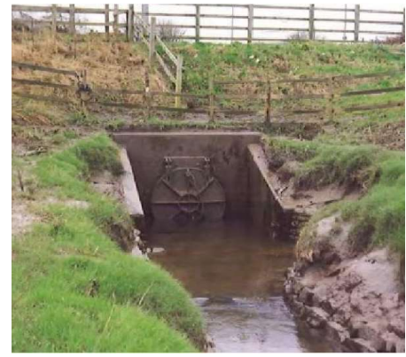
Existing north headwall
