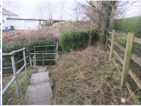
Existing south headwall
